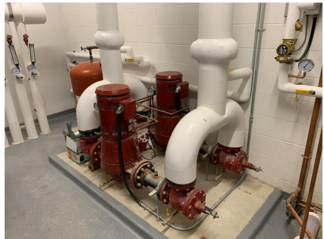
Figure 3: Dual Pump Geothermal Exchange System
