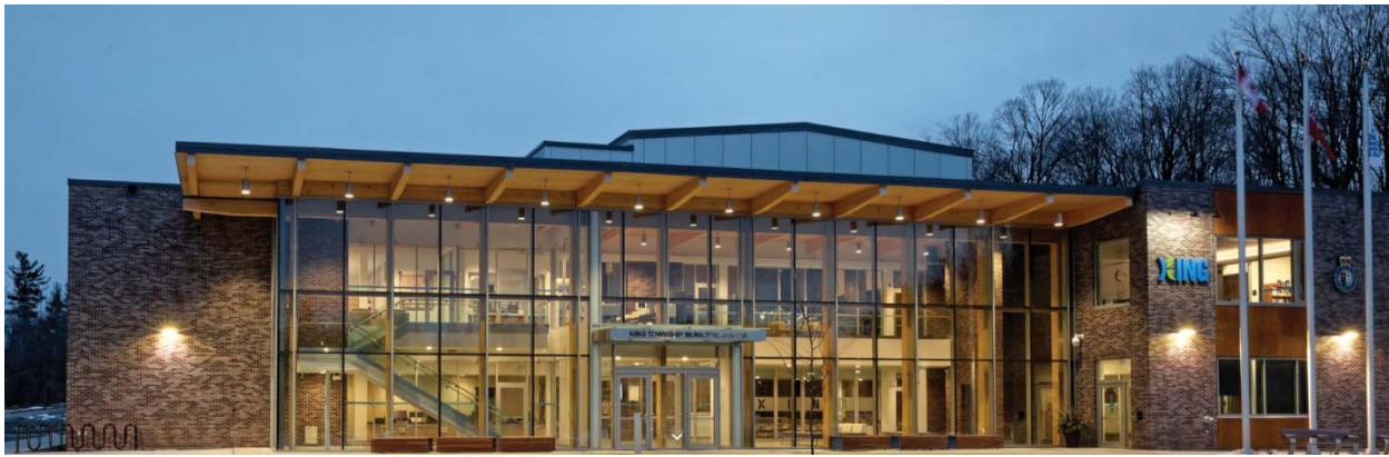
King Township Municipal Centre (KTMC)
