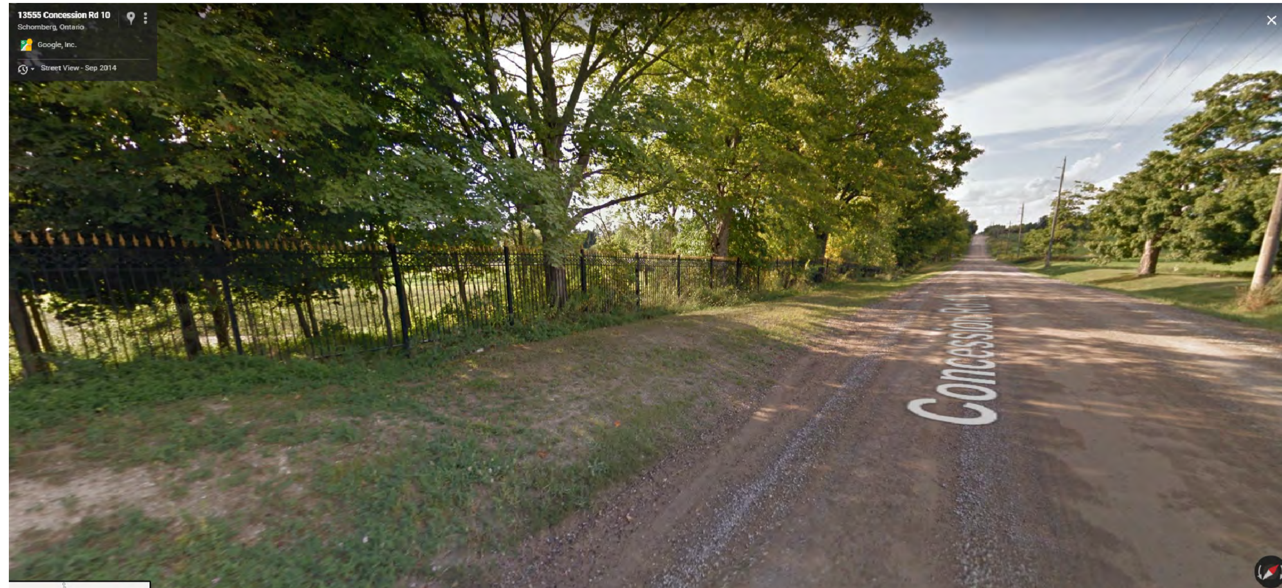
EXISTING WROUGHT IRON FENCE ALONG WEST PROPERTY LINE OF 10TH CONCESSION
